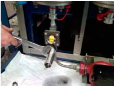
The compact sized MMT162 is easy to install to a T-piece of oil piping in a TRANSEC Unit.
