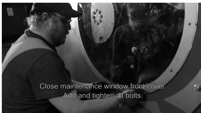
Figure 43. Closing the maintenance window
