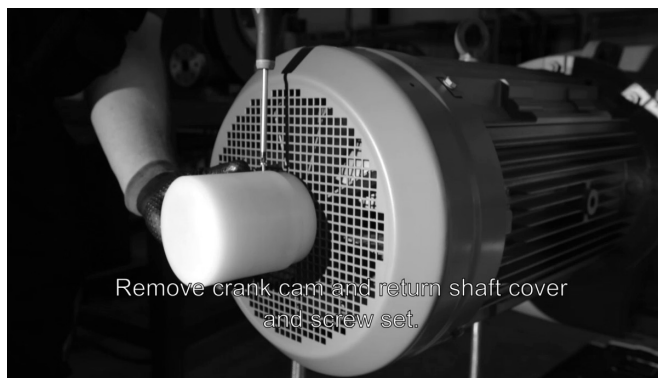
Figure 44. Installing the shaft cover
