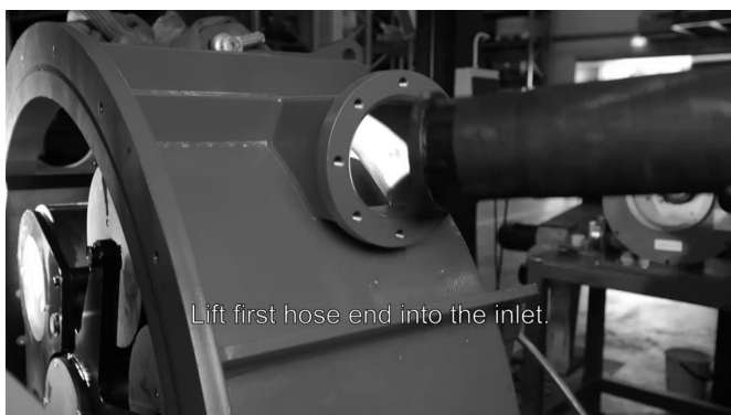
Figure 23. Installing the hose 1
