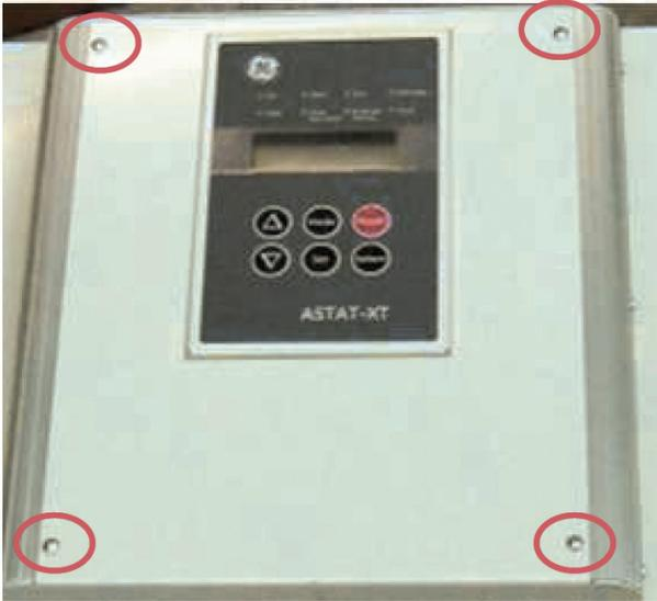
4. Remove 4 screws holding display unit.
