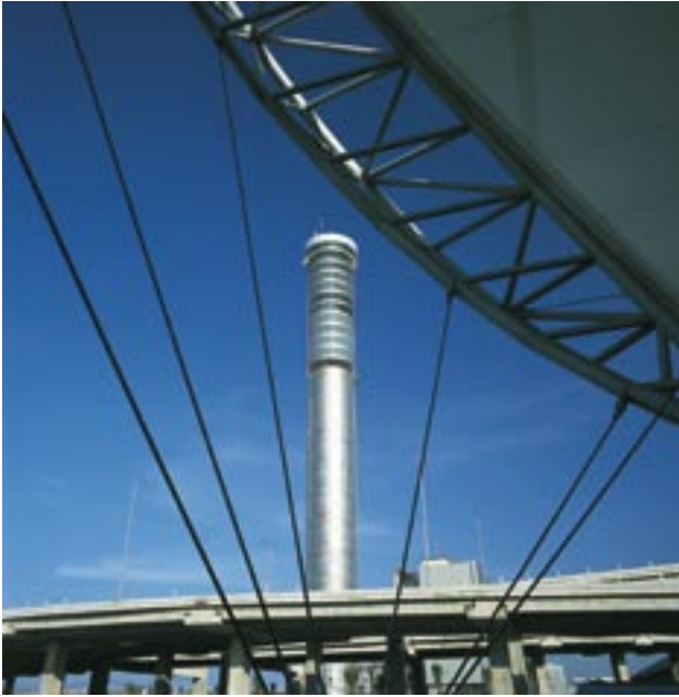
The Second Bangkok International Airport (SBIA) has the world's tallest control tower (132.2 m). Copyright: Tourism Authority of Thailand News Room, www.TATnews.org.
