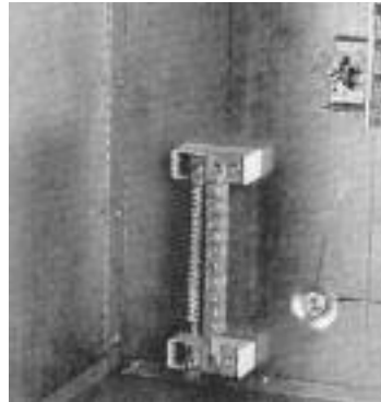
Isolated ground kit when required is field installed on either side
