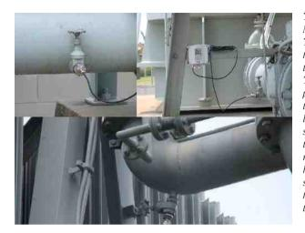
The probes of the Vaisala MMT338 Moisture and Temperature Transmitters for Oil are installed along the oil cooling circulation. The sensor at the top provides real-time data on temperature and moisture level, while the bottom sensor shows by how much the oil cools down in the radiator and how much higher the relative moisture saturation of oil is as it flows back into the transformer tank.
