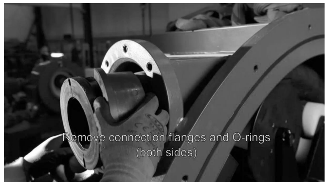
Figure 15. Removing the connection flanges and O-rings
