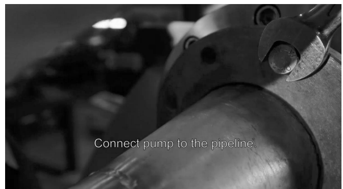
Figure 45. Connecting the pump to pipeline
