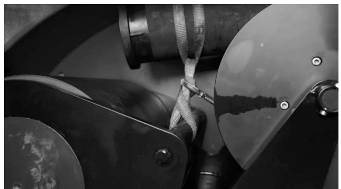
Figure 26. Installing the hose 4
