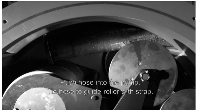
Figure 25. Installing the hose 3
