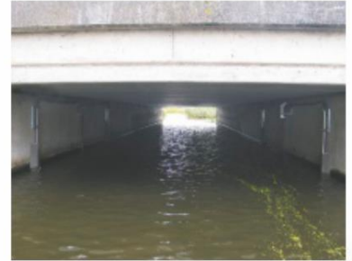
View of measurement place
